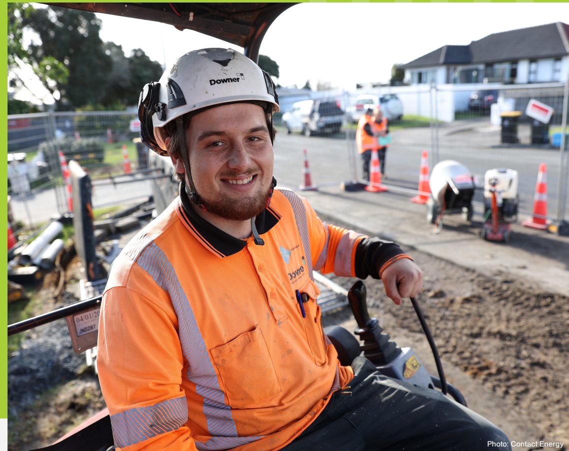
Photo: Contact Energy
