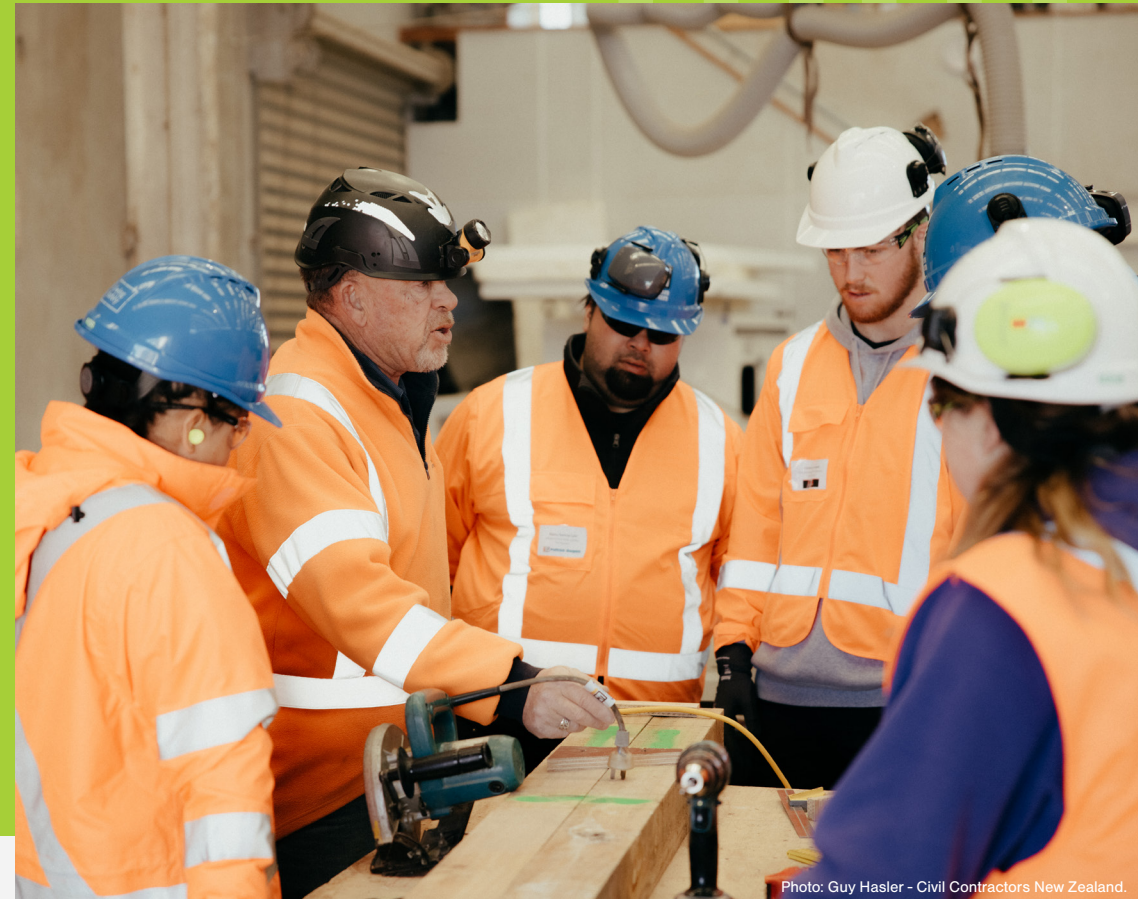
Photo: Guy Hasler - Civil Contractors New Zealand.
